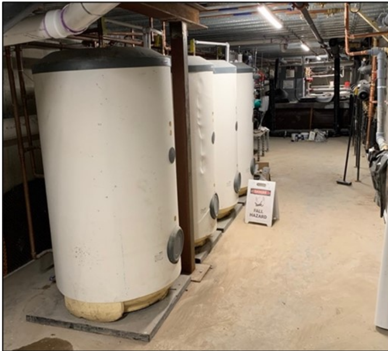
Figure 6. Photo of the DHW Tanks in Basement
