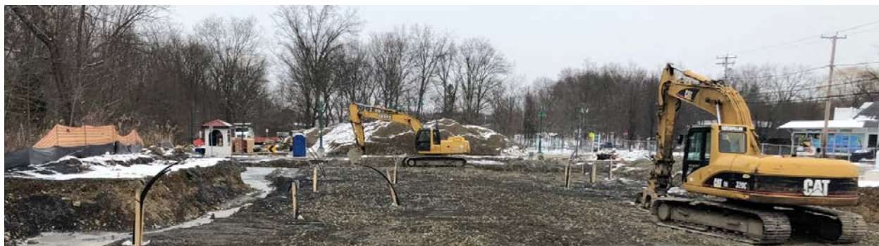
Figure 4. Photo of the Vertical Bores Installed Before Building Construction (the bores used only 15% of the building footprint)
